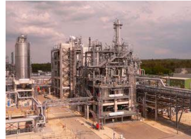
Lyondell Basell in Wesseling, Germany
